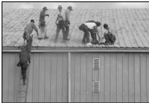
Amish putting the roof on the new IBT.
